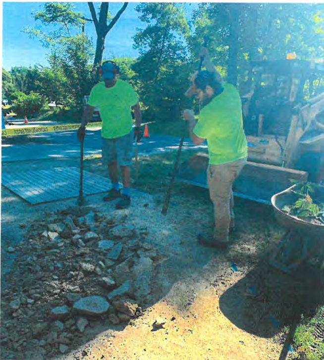
Path construction at Pondview Park
