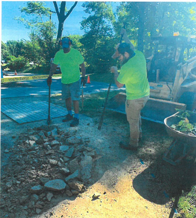
Path construction at Pondview Park
