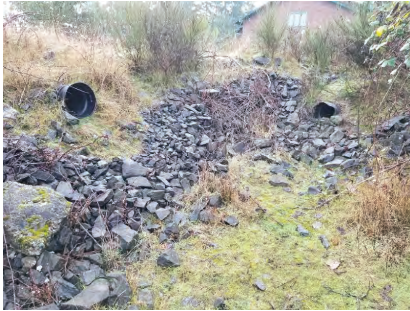
Photo 15. View Direction: South Viewing the outfall pipes at the south end of the upslope stormwater ditch. The pipe on the left conveys water to the eastern ditch along at the bottom of the slope. The pipe on the right conveys stormwater to the municipal stormwater sewer system.
