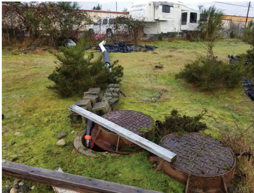
Photo 10. View Direction: Northwest Viewing a fifth-wheel trailer (background) and the trailer's gray water sanitary waste discharge pipe in the sanitary sewer manhole (foreground).
