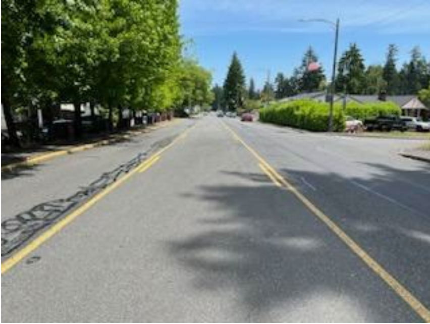
Figure 5. Regents Blvd (West) Grind and Overlay with ADA and pedestrian upgrades
