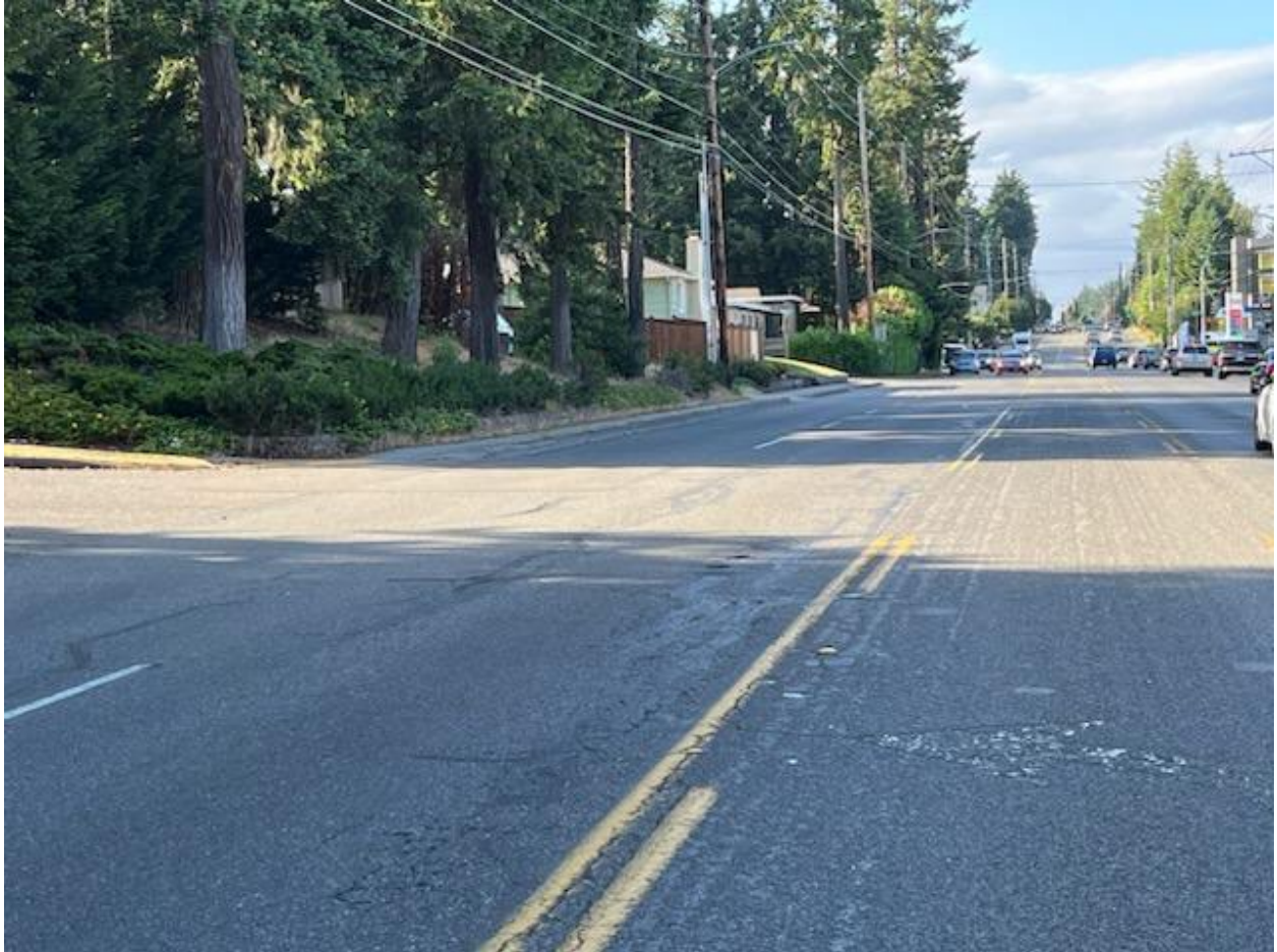
Figure 1. South Orchard St: Grind and Overlay with ADA upgrades - TIB Funded Grant
