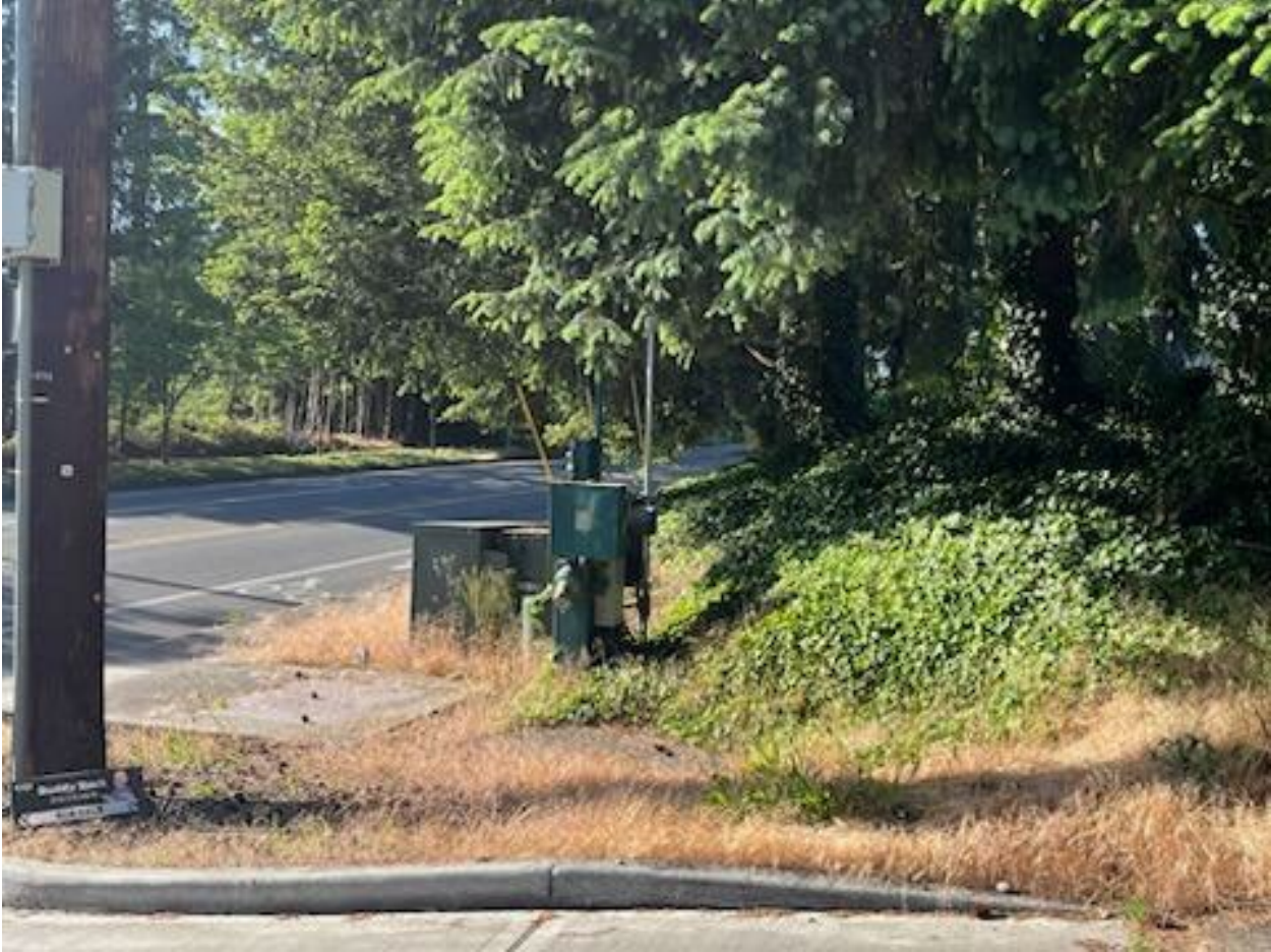
Figure 2. 44 th St W. Sewer Lift Station upgrade
