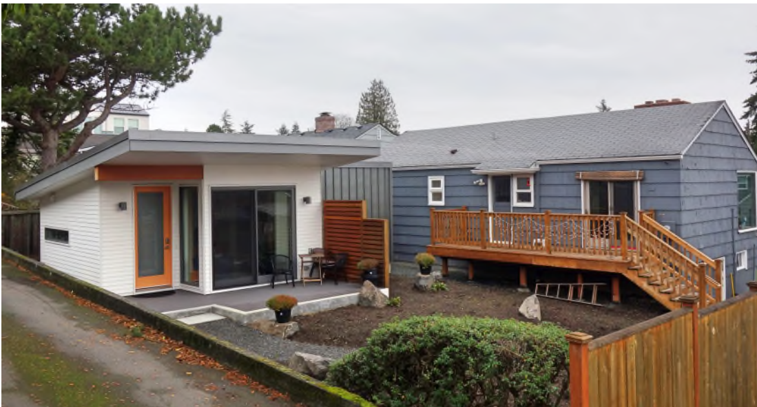
ADU in the Wedgewood neighborhood of Seattle. Credit: Pam MacRae, Sightline Institute . Used with permission.
