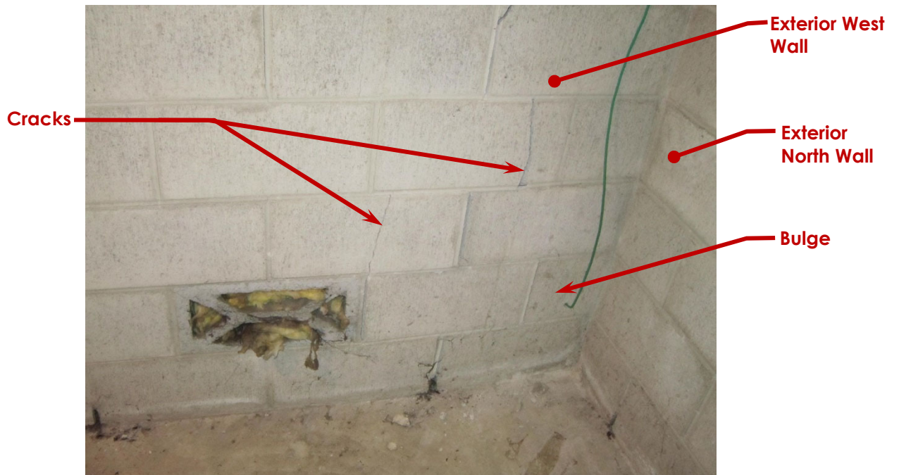
Photo 30 – Old Transformer Room Northwest Corner, Bottom
