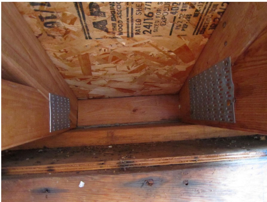
Photo 8 – Truss End Connection (Looking East)
