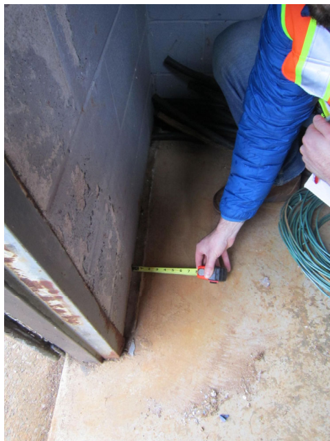
Photo 16 – South Entry Interior Face
