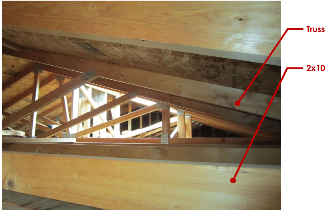
Photo 5 – Roof Trusses (Looking North)
