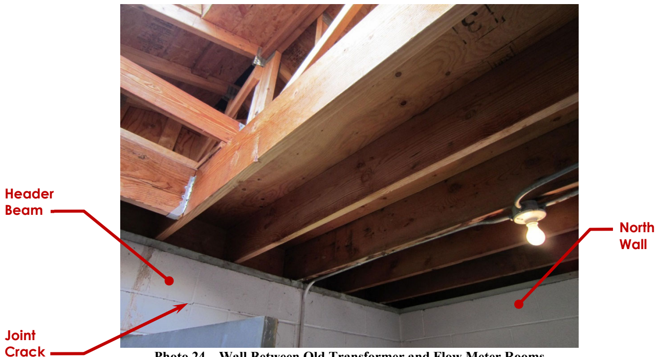
Photo 24 – Wall Between Old Transformer and Flow Meter Rooms (Looking Northwest)
