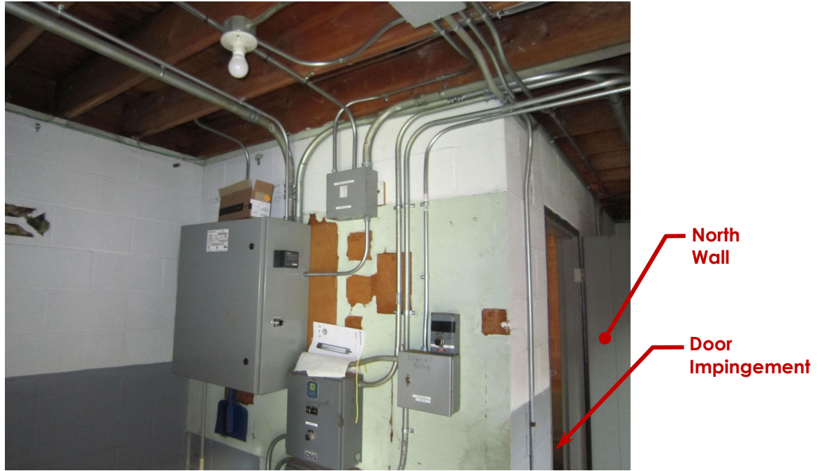
Photo 25 – Control Room North Wall (Looking Northwest)
