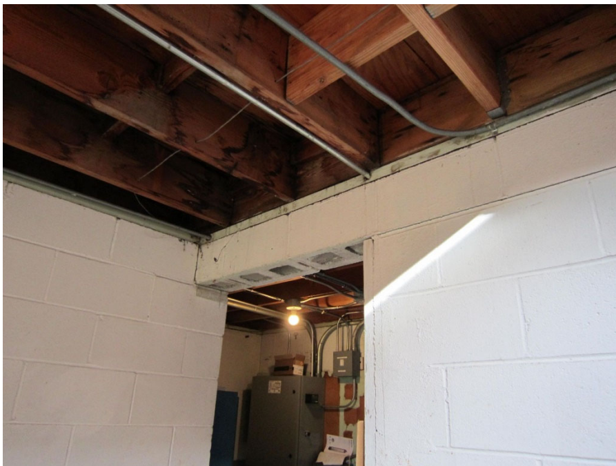
Photo 20 – Chlorine Pump Storage Room North Wall (Looking Northwest)
