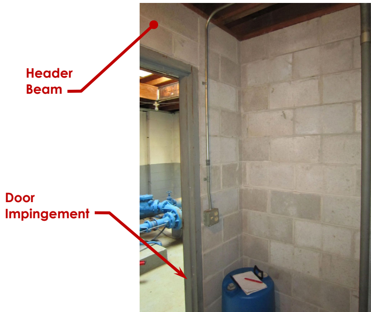
Photo 26 – Southwest Corner of Old Transformer Room
