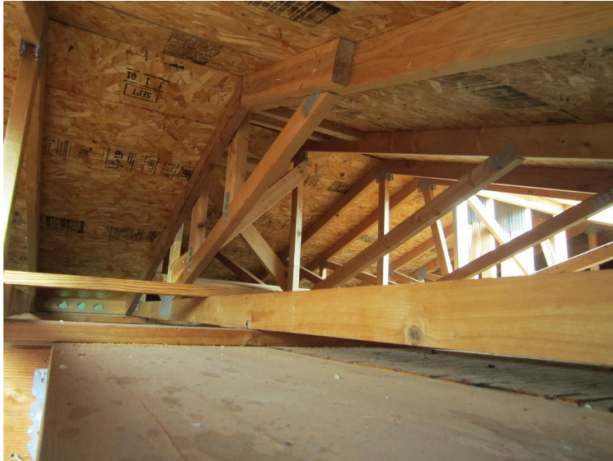
Photo 7 – Roof Trusses (Looking East)
