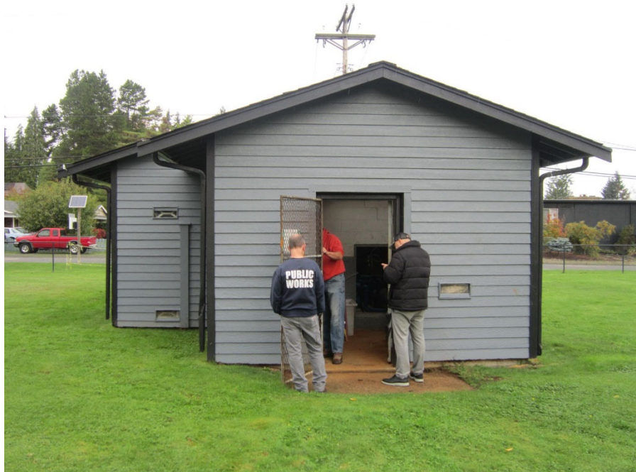
Photo 3 – South Face of Building
