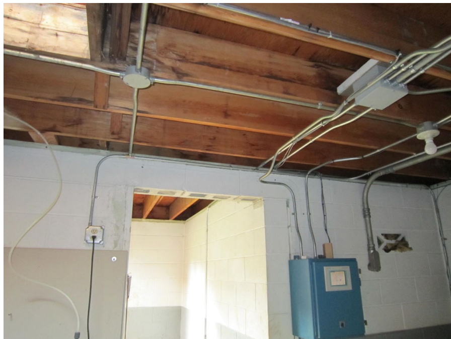
Photo 22 – Flow Meter Room South Wall (Looking South)
