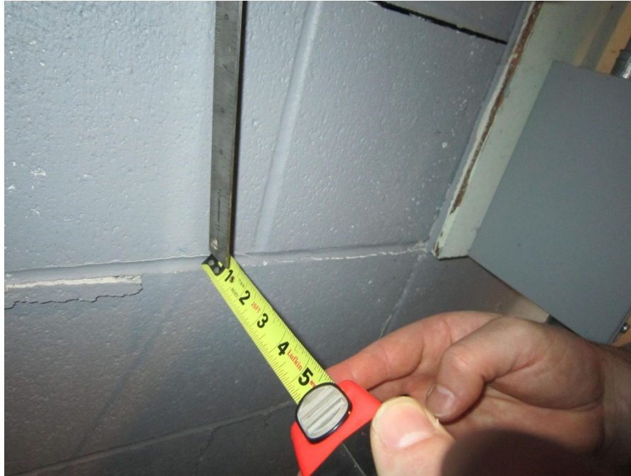
Photo 19 – Control Room North Wall (Northwest Corner)
