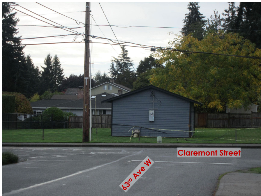
Photo 2 – North Face of Building
