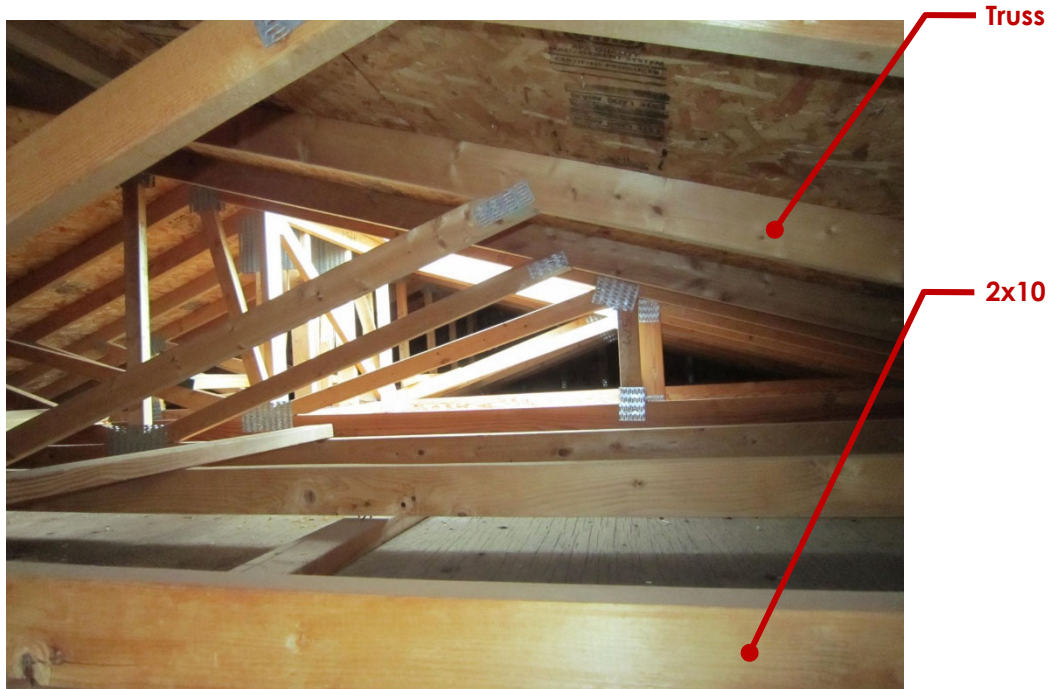
Photo 6 – Roof Trusses (Looking North)
