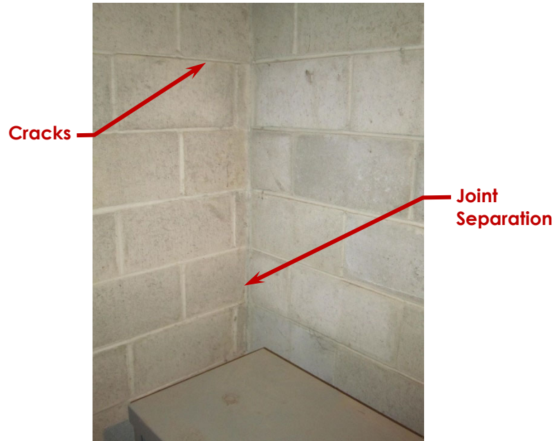
Photo 31 – Old Transformer Room Northeast Corner, Top
