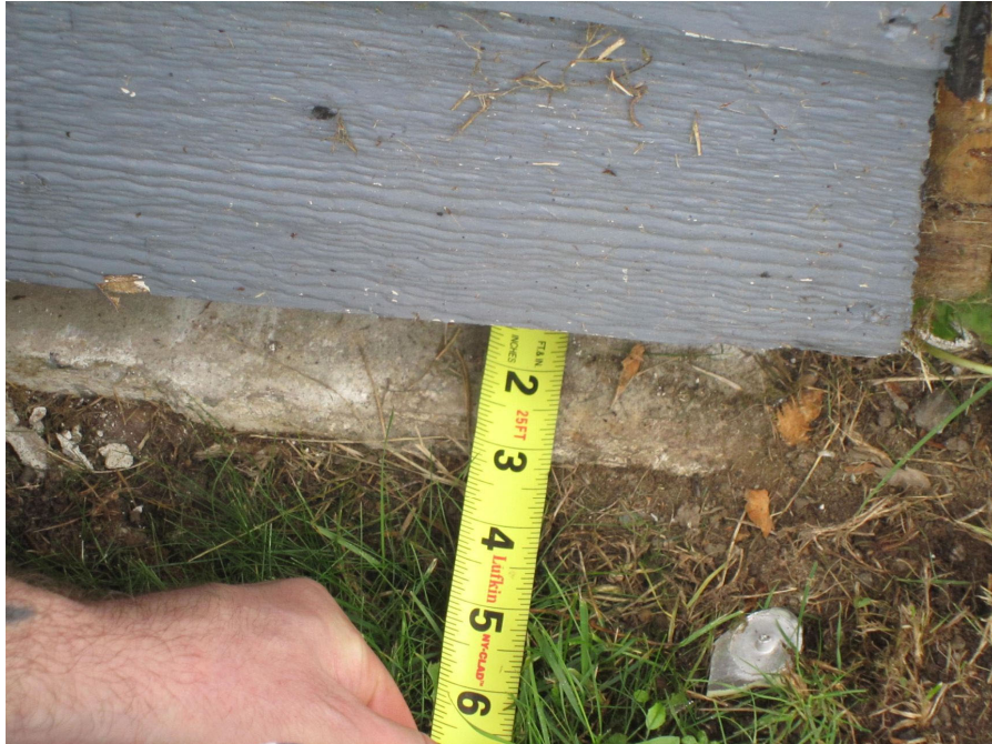
Photo 11 – Northwest Building Corner Base
