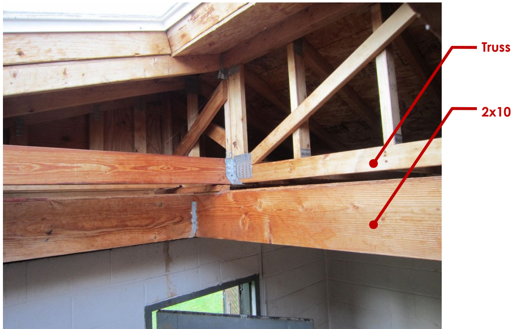
Photo 4 – Roof Trusses (Looking Southeast)
