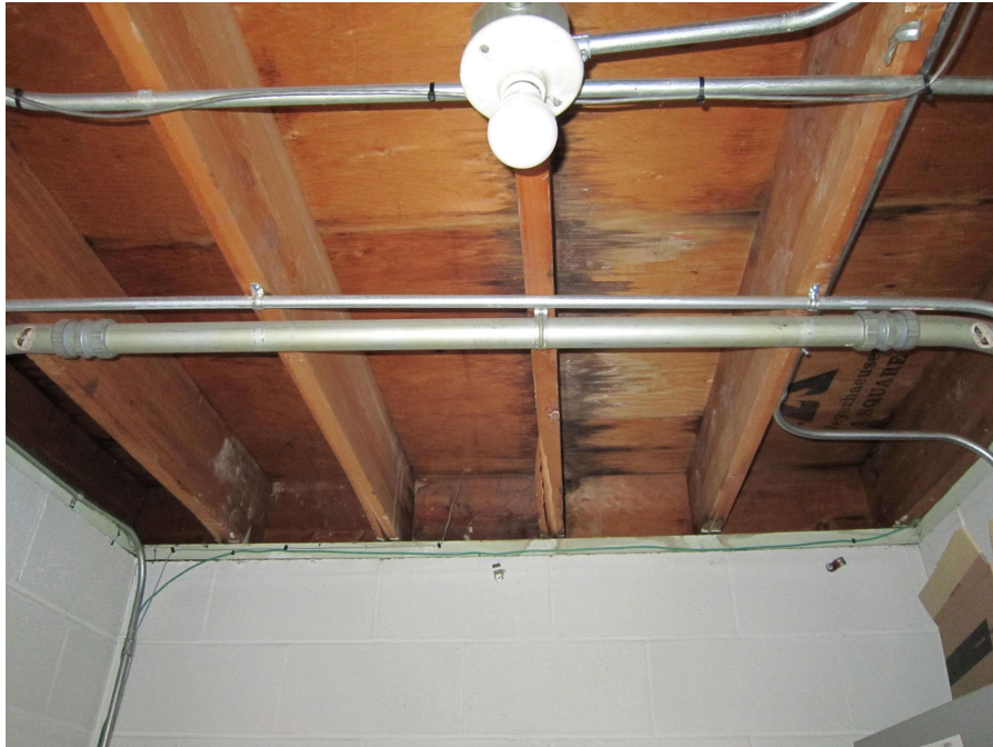
Photo 23 – Ceiling of Control Room (Looking West)
