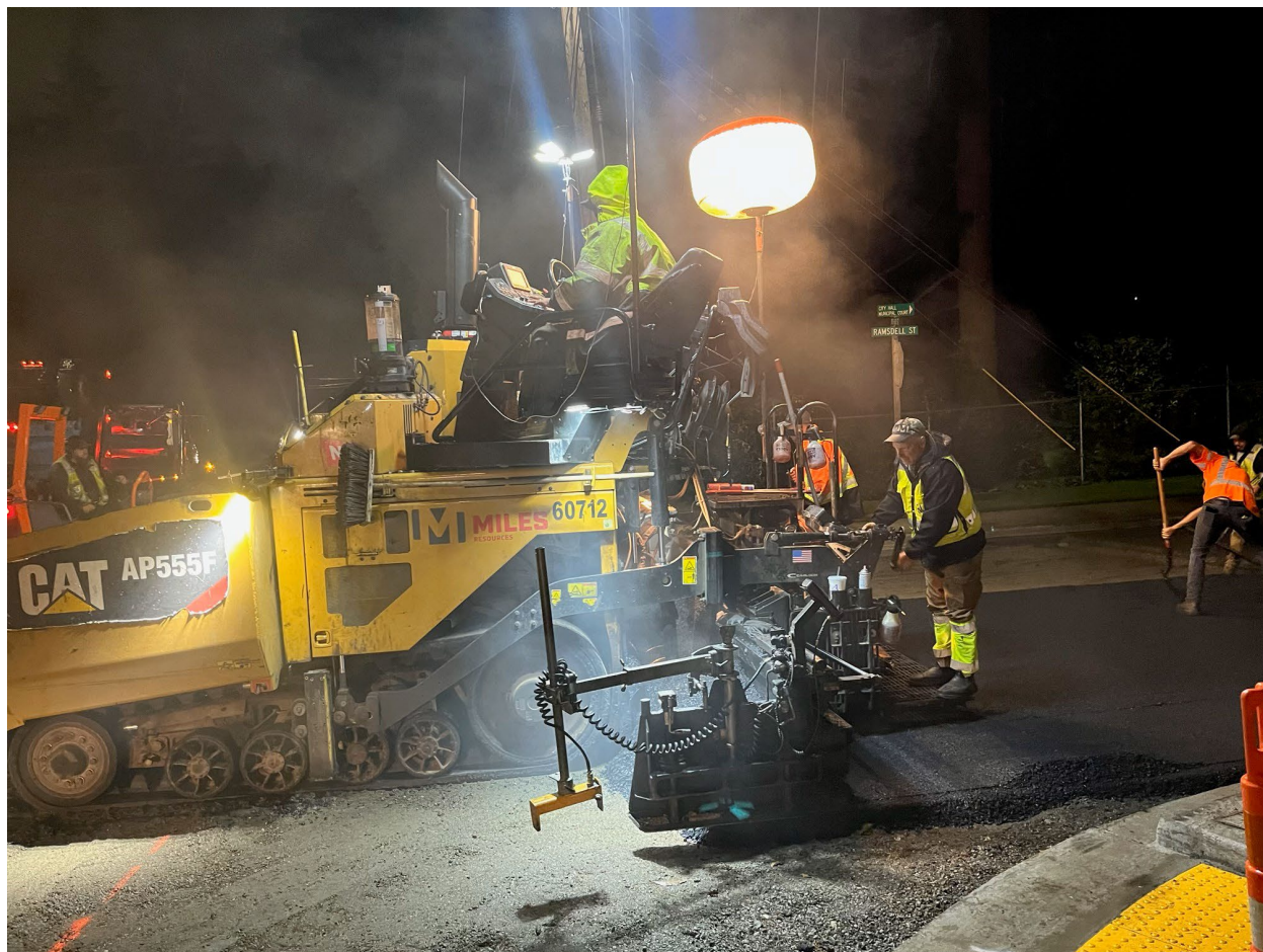
Orchard Boulevard Grind & Overlay Work
