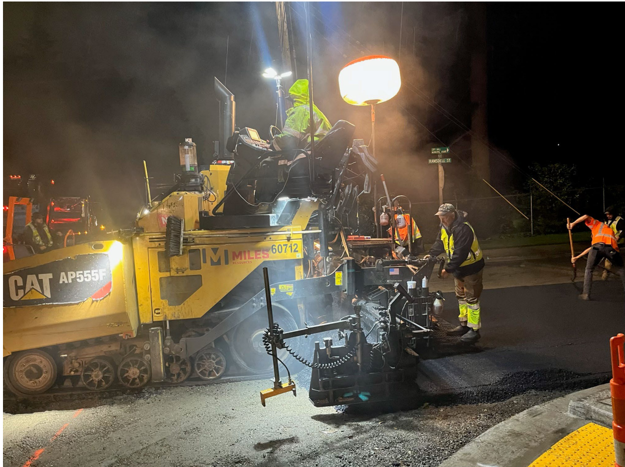
Orchard Boulevard Grind & Overlay Work
